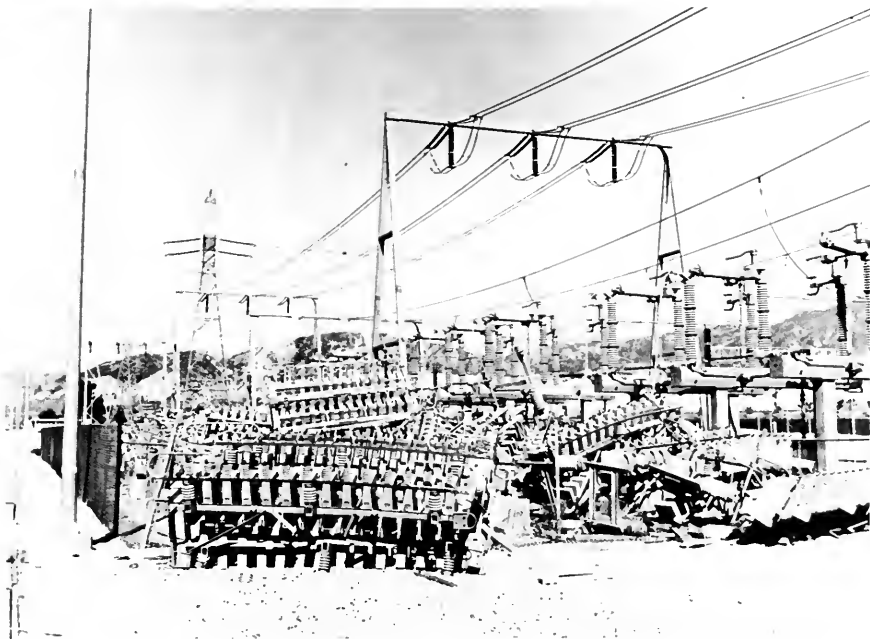
Photo 26. Sylmar Converter Station. Toppled filter capacitor banks. Las Angeles Department of Water and Power photo.
